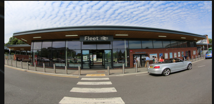
Fleet Mainline Railway Station
