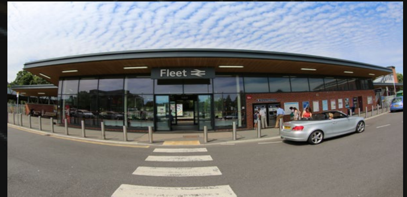
Fleet Mainline Railway Station
