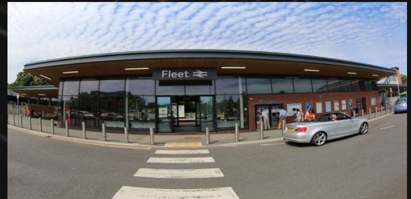
Fleet Mainline Railway Station
