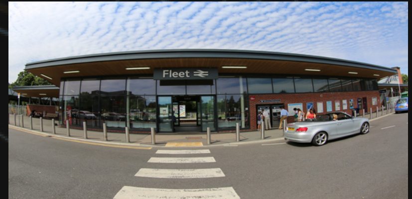
Fleet Mainline Railway Station
