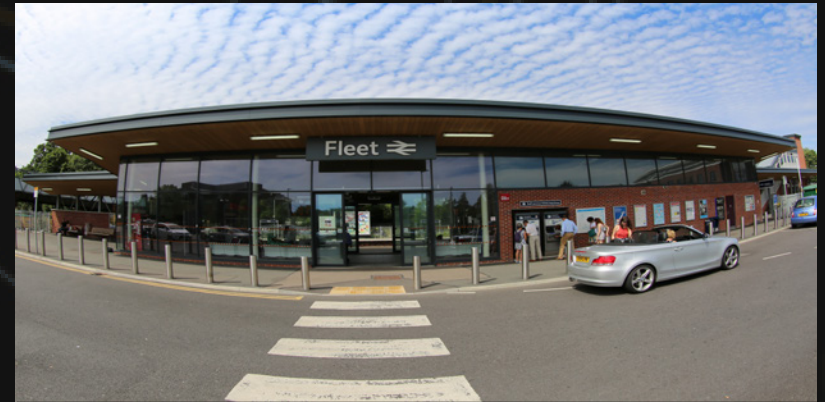
Fleet Mainline Railway Station
