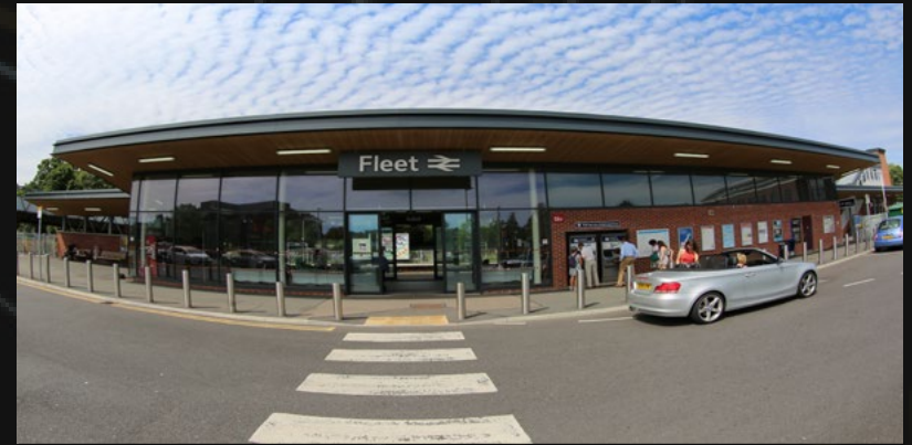
Fleet Mainline Railway Station
