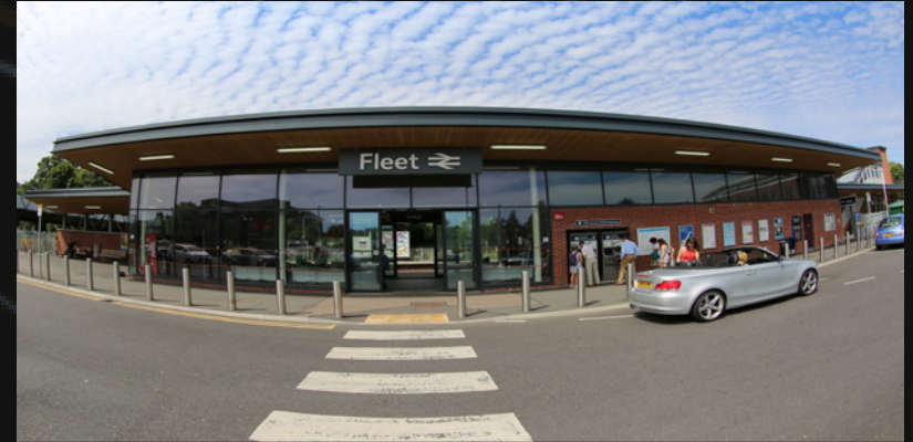
Fleet Mainline Railway Station
