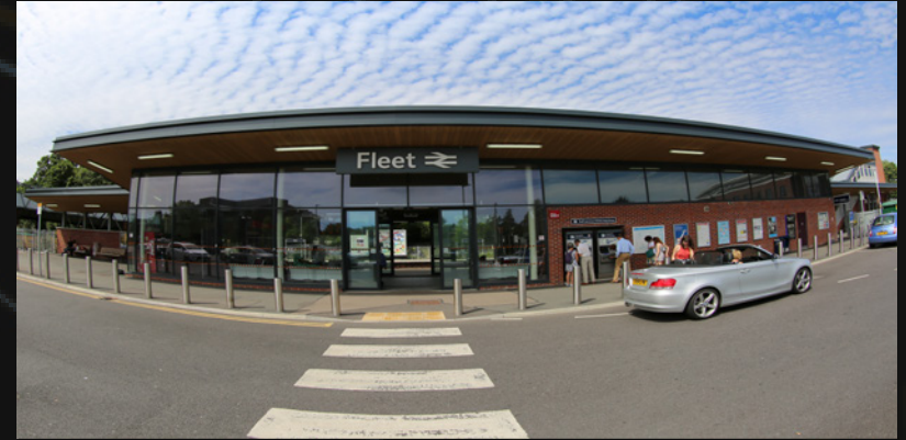
Fleet Mainline Railway Station
